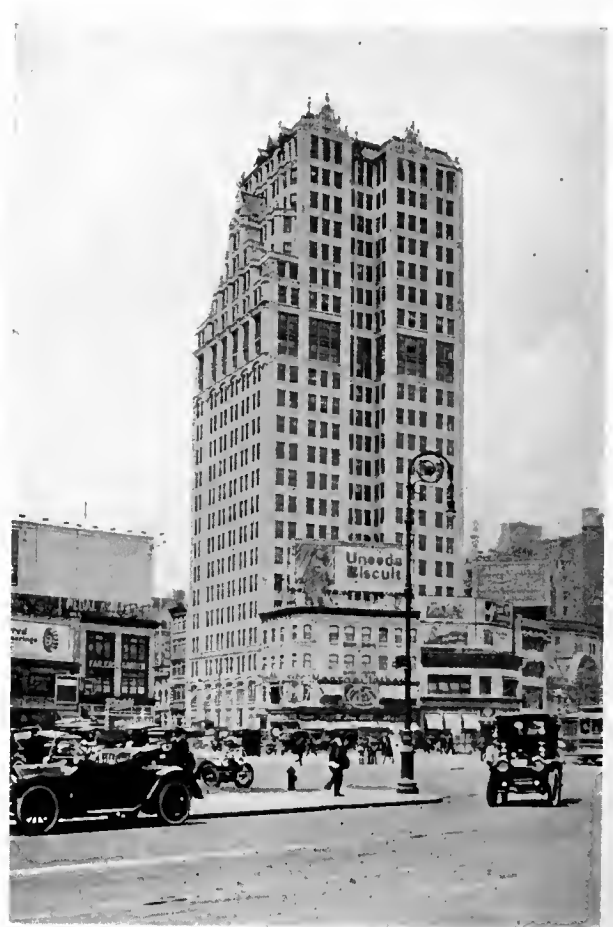
FIG. 2. GOTHAM NATIONAL BANK BUILDING, COLUMBUS CIRCLE, NEW YORK
